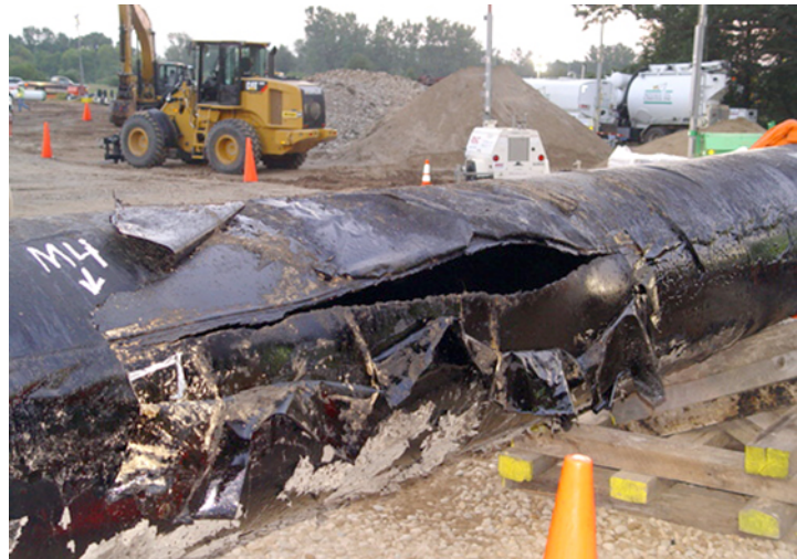
This pipe was inspected and considered safe but eventually leaked 20,000 barrels of oil into the Kalamazoo River
